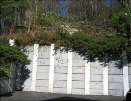
MAINTENANCE CREWS WEEDS AND CLEANED THE ENTIRE AREA SURROUNDING THE PROPERTY, LEAVING A MUCH NEATER APPEARANCE
