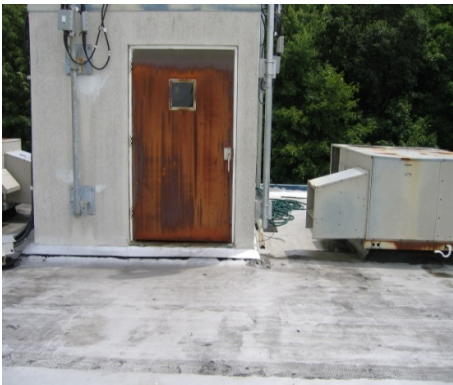
THE HEAVILY RUSTED DOOR ON THE ROOF WAS SANDED AND PAINTED TO PROTECT IT FROM THE HARSH ELEMENTS. AND A NEW LOCK AND CLOSING DEVICE WERE INSTALLED TO MAKE THE ROOF ACCESS MORE SECURE
