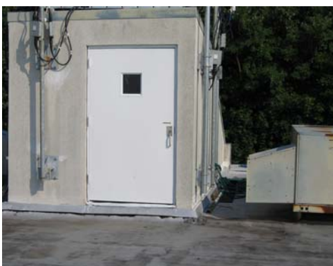
THE HEAVILY RUSTED DOOR ON THE ROOF WAS SANDED AND PAINTED TO PROTECT IT FROM THE HARSH ELEMENTS. AND A NEW LOCK AND CLOSING DEVICE WERE INSTALLED TO MAKE THE ROOF ACCESS MORE SECURE
