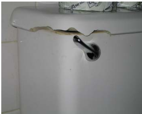
THE CRACKED TOILET TANK LID IN THE THIRD FLOOR MEN'S RESTROOM WAS REPLACED WITH A NEW ONE
