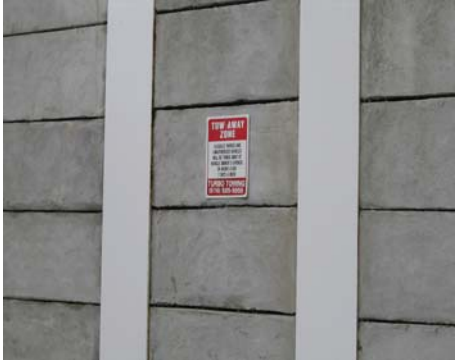
ALL OF THE STEEL COLUMNS ON THE RETAINING WALLS IN THE REAR PARKING LOT WERE SCRAPED AND PAINTED TO PROTECT THEM FROM THE ELEMENTS AND TO ENHANCE THE APPEARANCE OF THE PROPERTY
