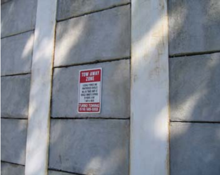
ALL OF THE STEEL COLUMNS ON THE RETAINING WALLS IN THE REAR PARKING LOT WERE SCRAPED AND PAINTED TO PROTECT THEM FROM THE ELEMENTS AND TO ENHANCE THE APPEARANCE OF THE PROPERTY
